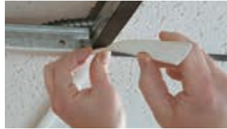
Applying GridMax Over T-bar Suspension Grid System
